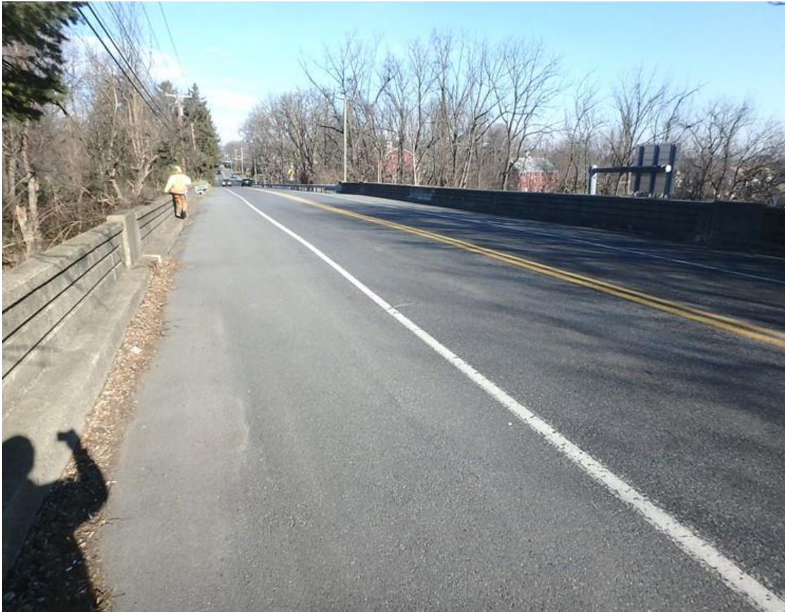
Photo #1 : SR 2028/BRKEY 28745 - View of bridge deck. Photo Date: 1/12/2021.
