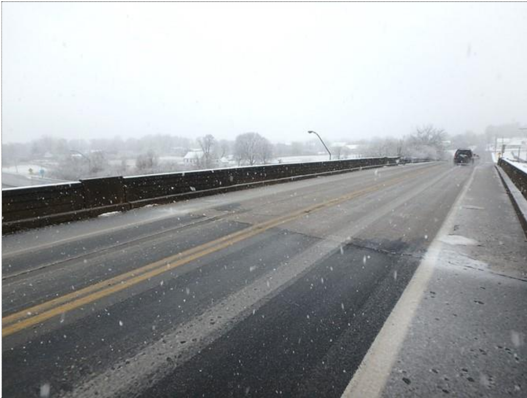
Photo #1 : SR 2028/BRKEY 28744 - View of bridge deck. Photo Date: 12/14/2020.
