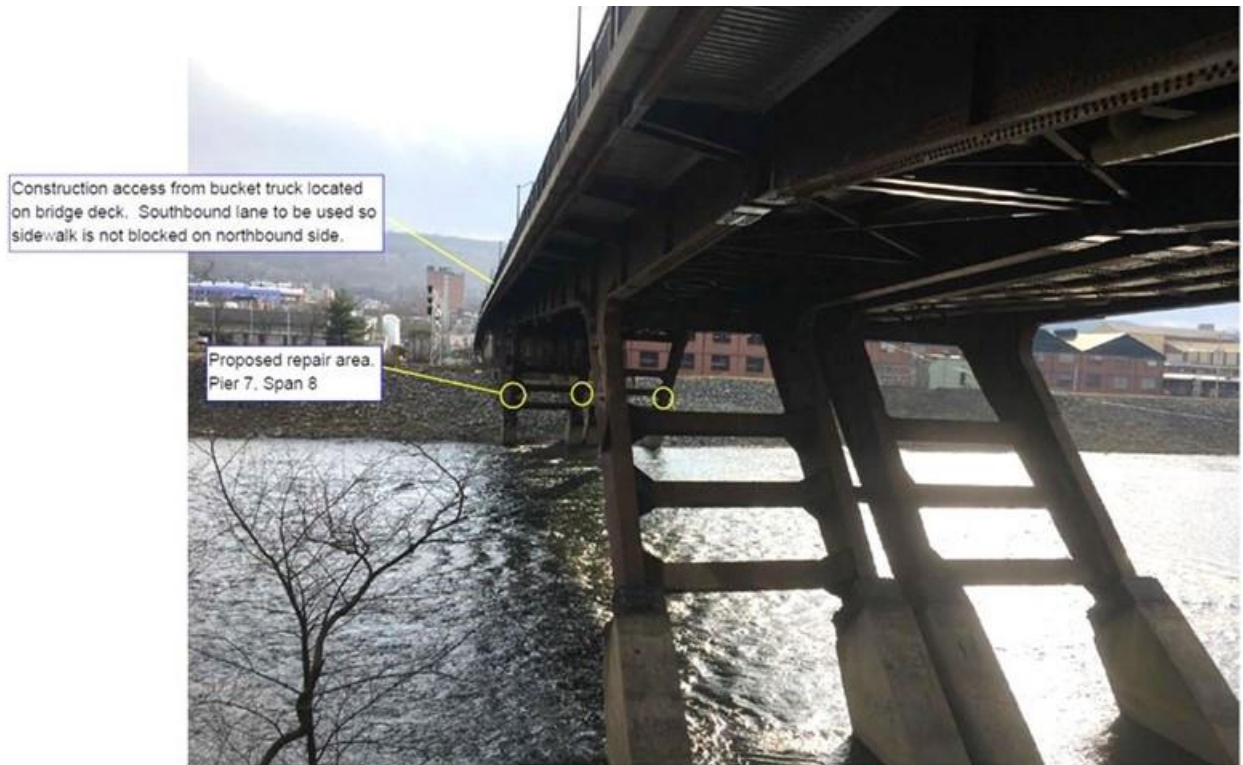
Photo #1 : SR 3011/BRKEY 28761 - View of Pier 7 repair locations. Photo Date: 12/14/2020.
