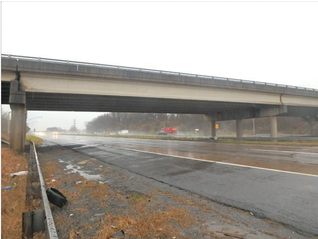
Photo #2 : SR 3020/BRKEY 28771 – Elevation view of bridge. Photo Date: 12/14/2020.
