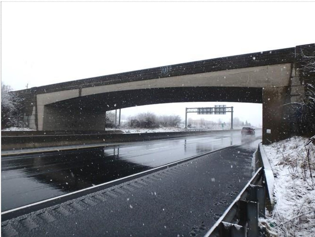
Photo #2 : SR 2028/BRKEY 28744 - Elevation view of bridge. Photo Date: 12/14/2020.
