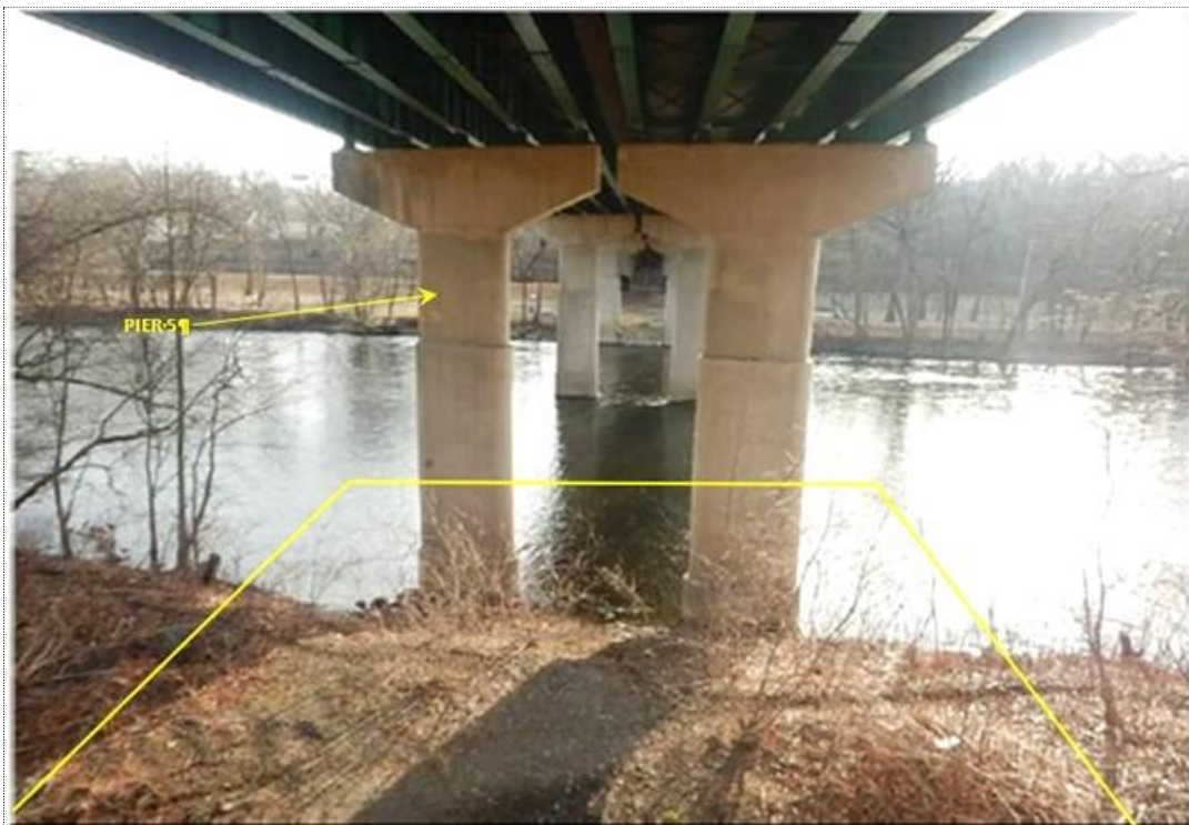
Photo #2: SR 2012/BRKEY 28723 - View of work area (Pier 6) looking east toward Lehigh River. Photo Date: 2/12/2020.
