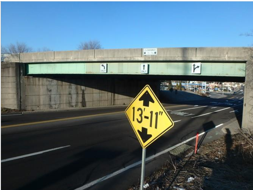
Photo #2 : SR 0022/BRKEY 28481 - Elevation view of bridge. Photo Date: 1/12/2021.
