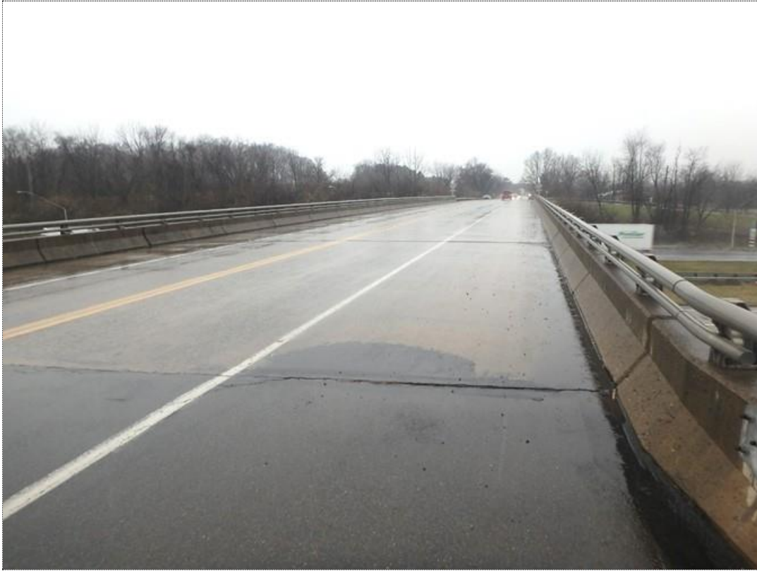
Photo #1 : SR 3020/BRKEY 28771 – View of bridge deck. Photo Date: 12/14/2020.
