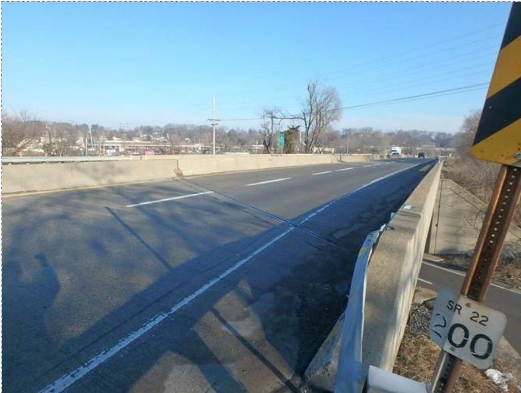
Photo #1 : SR 0022/BRKEY 28481 - View of bridge deck. Photo Date: 1/12/2021.
