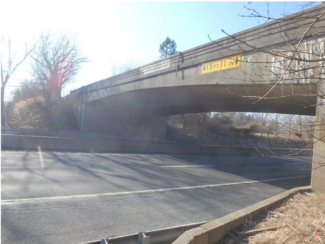
Photo #2 : SR 2028/BRKEY 28745 – Elevation view of bridge. Photo Date: 1/12/2021.
