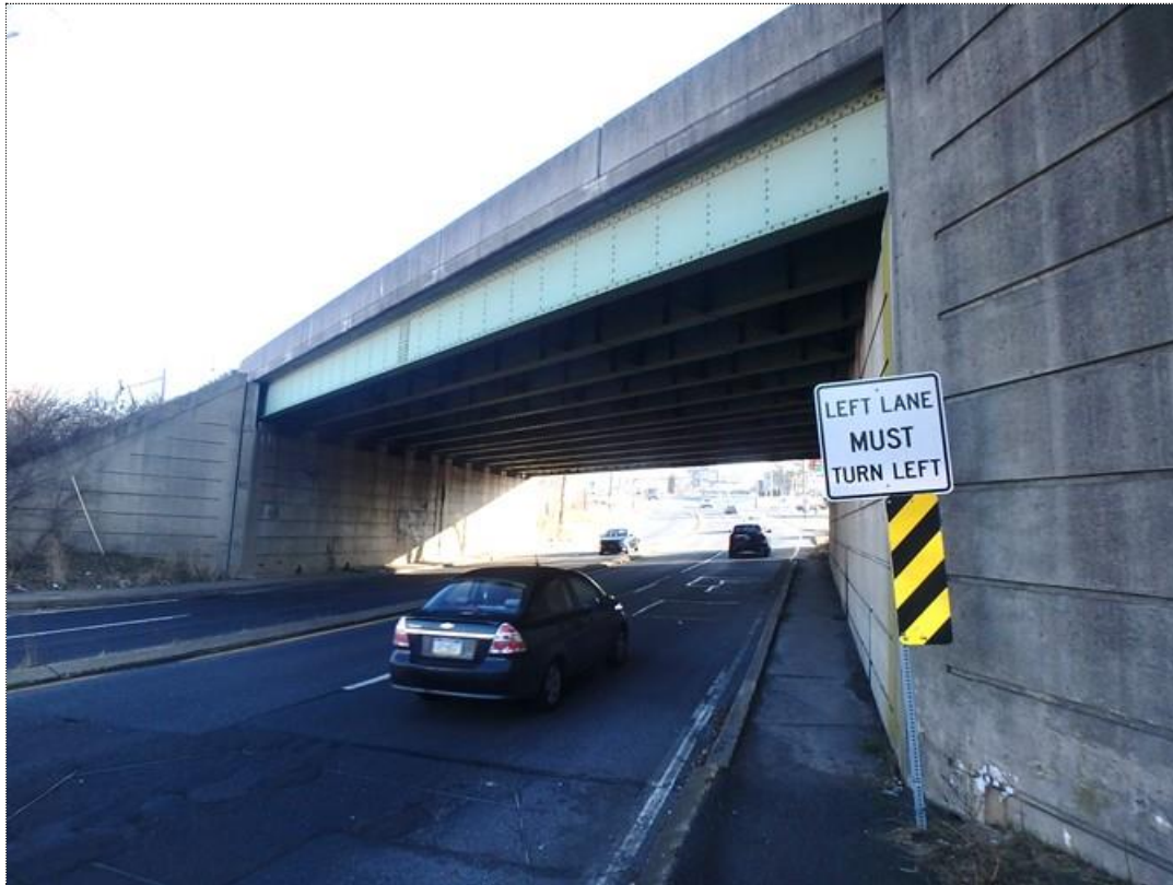
Photo #1 : SR 0022/BRKEY 28482 – Elevation view of bridge. Photo Date: 1/12/2021.
