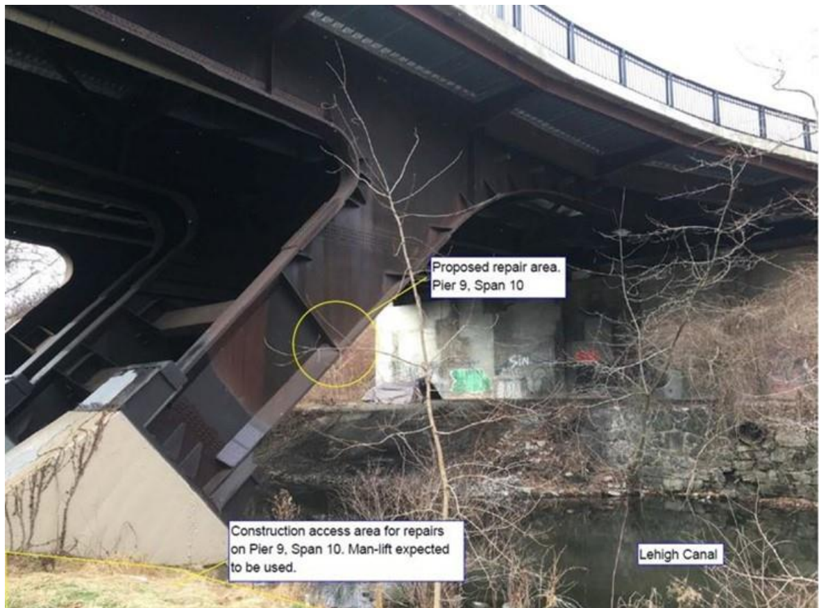
Photo #4 : SR 3011/BRKEY 28761 – Review of Pier 9 repair location. Photo Date: 1/19/2021.
