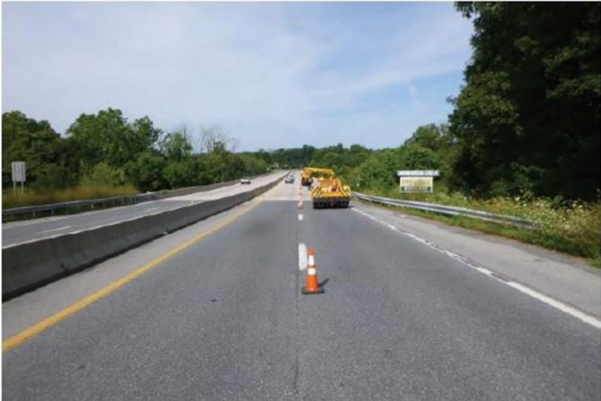
Photo #1 : SR 0145/BRKEY 39624 - View of bridge deck. Photo Date: 8/5/2019.
