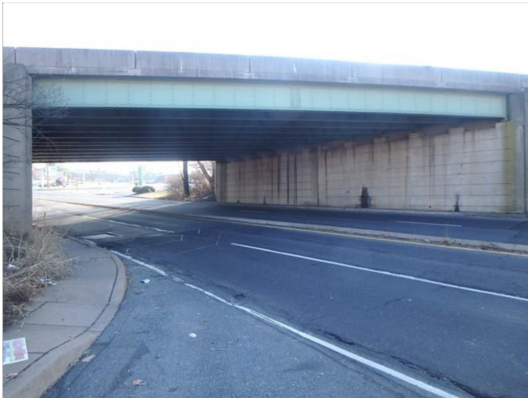
Photo #2 : SR 0022/BRKEY 28482 - Elevation view of bridge. Photo Date: 1/12/2021.
