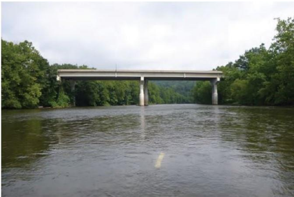
Photo #2 : SR 0145/BRKEY 39624 - Elevation view of bridge. Photo Date: 8/5/2019.
