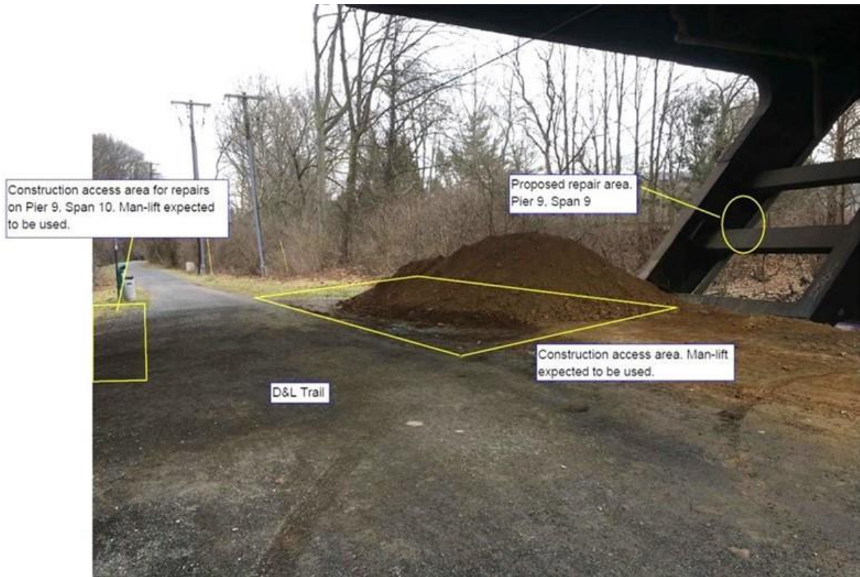
Photo #3 : SR 3011/BRKEY 28761 - View of Pier 9 repair location. Photo Date: 12/14/2020.
